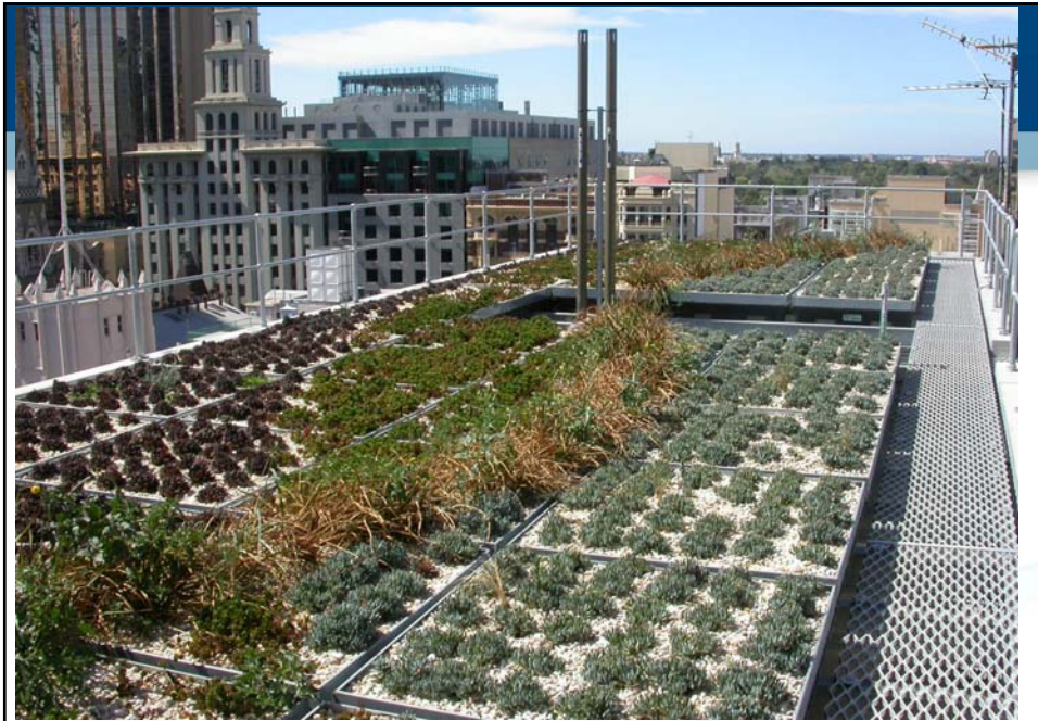
CH2 East Core Roof - February 2007
