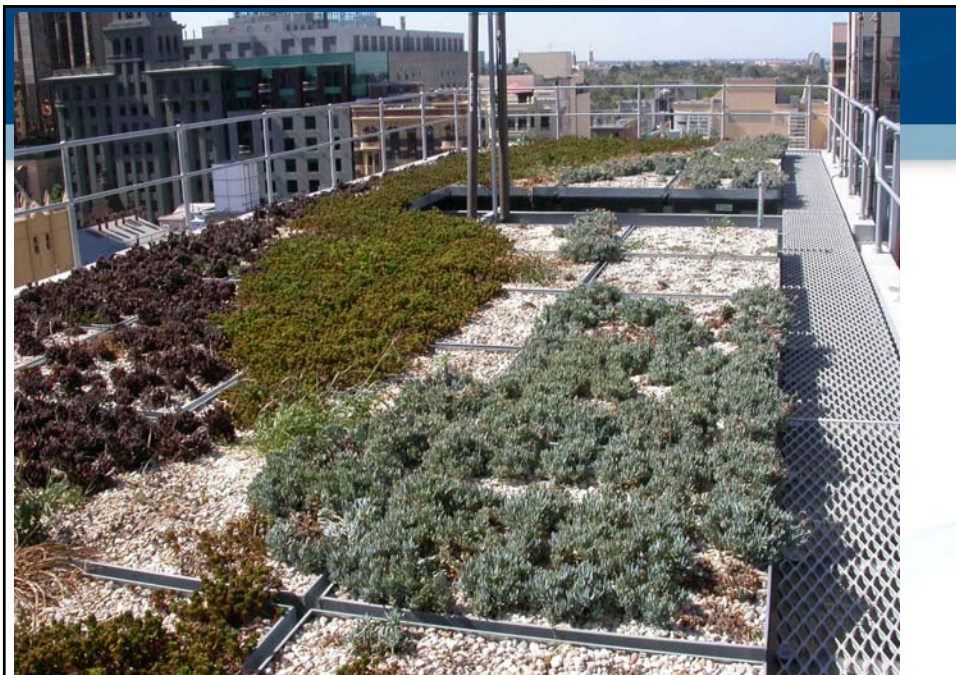
CH2 East Core Roof - February 2008
